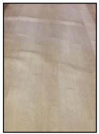
influence of a heat run under the floor causing a reaction with the underlayment and certainly not the reaction that the underlayment expanded like a dry sponge suddenly soaked with water.
