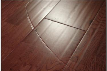
Gouge in Engineered Wood Floor
