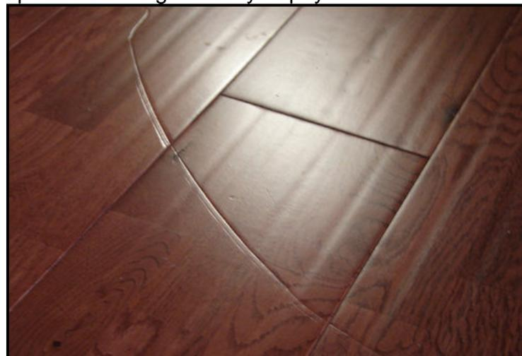
Gouge in Engineered Wood Floor
