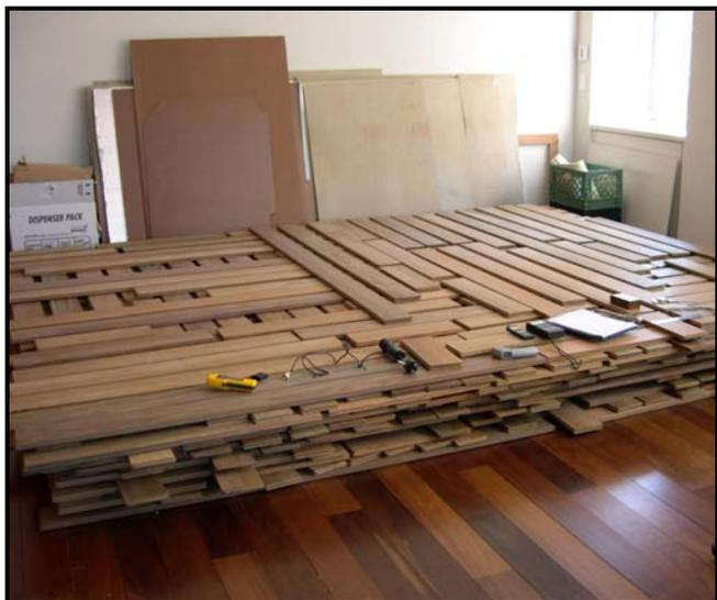
Wood flooring is, after all, still a tree but in board form and it will do the same things when made into boards used for flooring that it does in the forest. Wood can and will, expand, contract, warp and, as previously stated, dent, scratch and gouge. Wood flooring must be protected after installation to prevent damage to it that you cannot blame the
