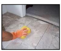
clean clear water prior to application. Pack the grout into the joints in a perpendicular motion, passing over the area to be grouted a minimum of three times. Let the joint stiffen which takes 15 to 30 minutes
