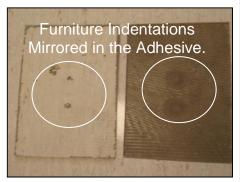
Heavier beds and heavier patients in health care environments, when statically positioned, that is stationary in one place, will compress the vinyl flooring and cause indentations. Hospital beds can weigh up to 600 pounds and if they have thin, sharp crowned wheels they can and will wreak havoc on vinyl flooring. Add to that a heavy patient in the bed and it's possible to exert over 1,000 pounds of pressure to the flooring material.
