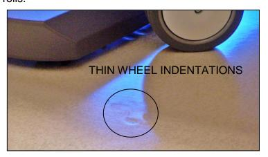
The products may have changed as well. As the industry strives to be green and improvements made to vinyl products along these lines, the ability to resist indentation may be compromised. And there may actually be a defect in the material that will allow it to be more susceptible to indentation.
