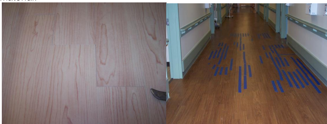
Shrunken LV Plank Over Abated Substrate
