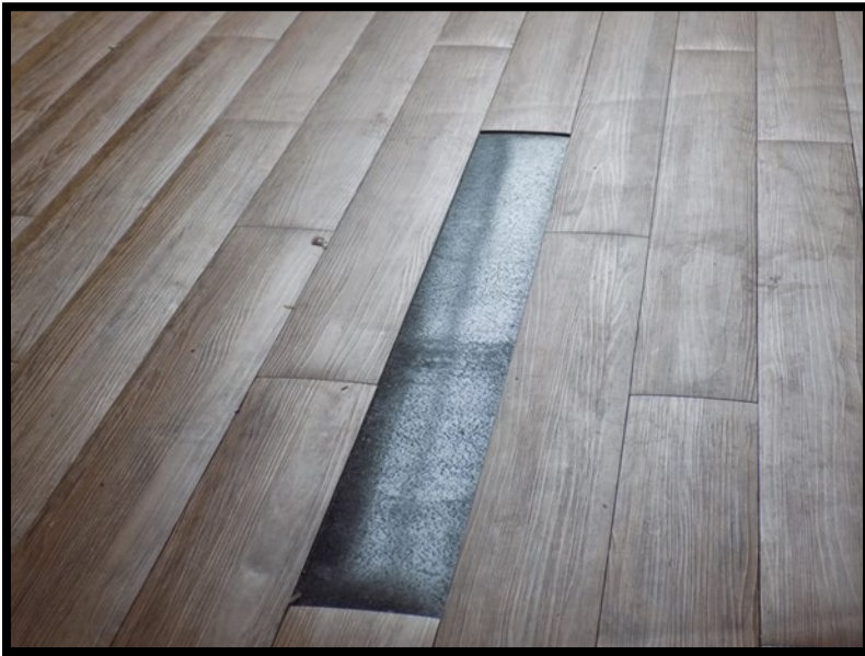
An example of the reaction between SBR crumb rubber underlayment and PVC vinyl plank.
