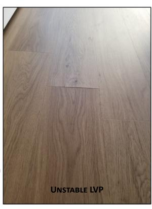
nesses of the components, slight cup or crown may be present. Wood moves only minimally along the length, so, expansion of the PVC in the length direction will cause the plank ends to lift. There are several variables that can cause this explanation to be invalid, but the majority of products with 0.5mm to 1.2mm veneers adhered to rigid PVC will exhibit the issues described.
