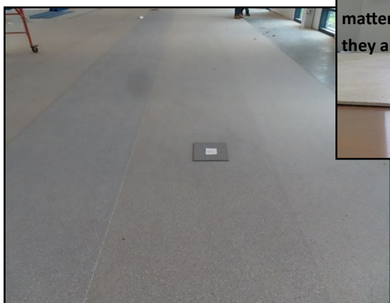
Three rolls of rubber flooring that are supposed to be the same for this project but every roll color shade varies.
