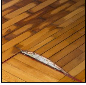
Inaccurate test results from leapfrogging could lead to bad decisions about when to install, and that could mean a costly flooring failure.
