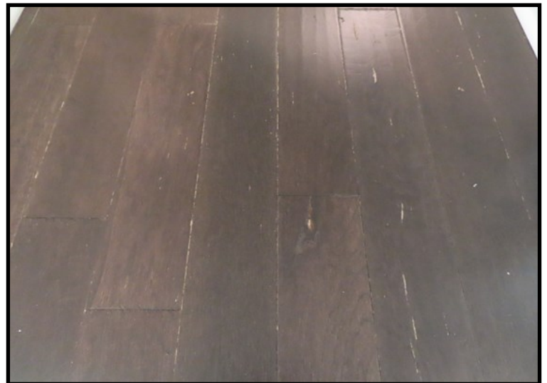
Wood flooring in luxury condos with the finish coming off. This was a very defective product involving a multi-million-dollar lawsuit that we won for our client. We went molecular on this one to prove the product was defective.
