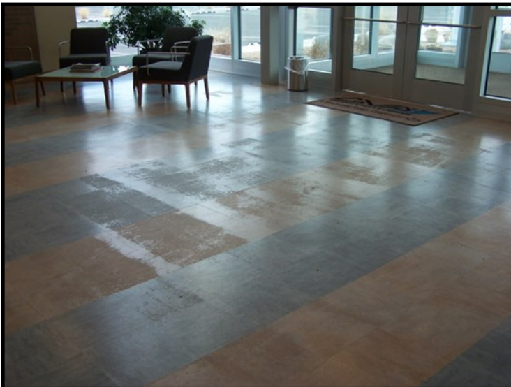
A natural flooring product with the surface finish wearing off. A new coating was applied that didn't work either.
