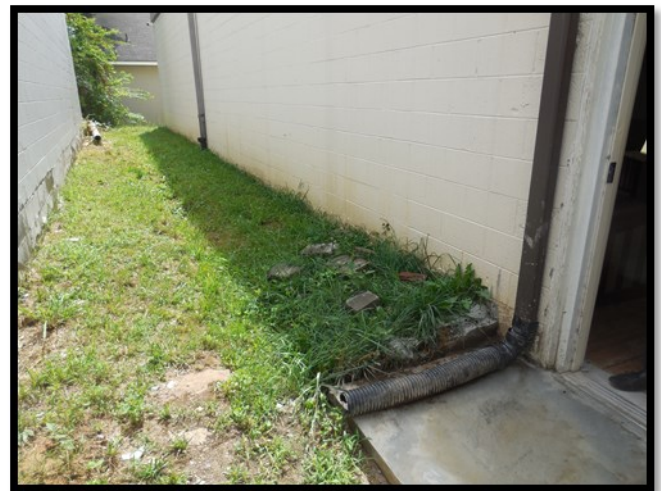
ALWAYS LOOK OUTSIDE PART OF THE SLAB IS ON GRADE AND PART BELOW DUE TO THE GRADING OF THE BUILDING
