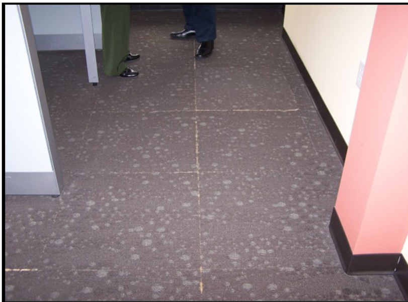
Moisture caused flooring failure. So much moisture that the adhesive is oozing out between the edges of the carpet tiles like lava from a volcano. This is the job mentioned that we developed a fix for.
