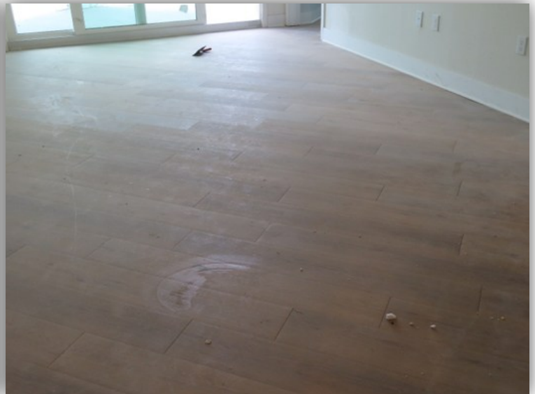
Shade variation in vinyl plank due to surface texture differences. All from the same run and boxes.
