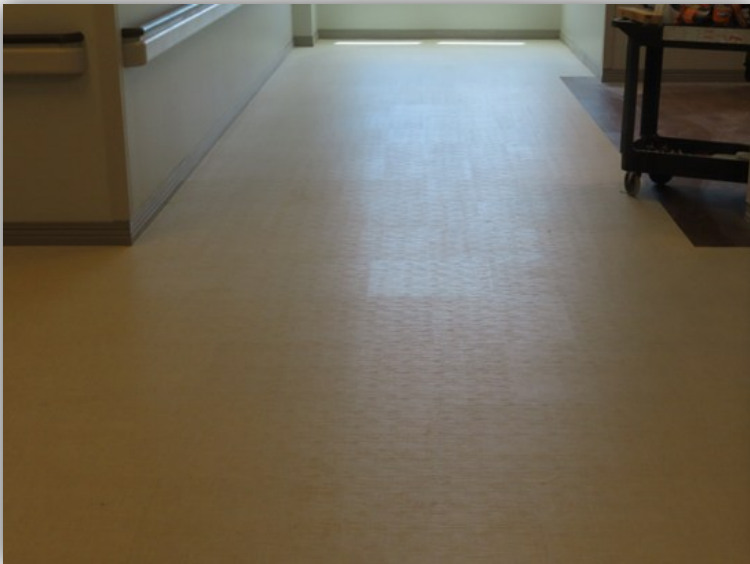
Shade, sheen and texture variation in vinyl tiles evident in streaming sunlight.
