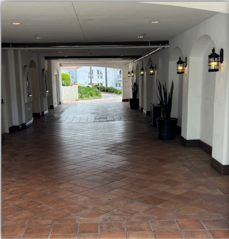
Ceramic tile shade variation from a distance.
