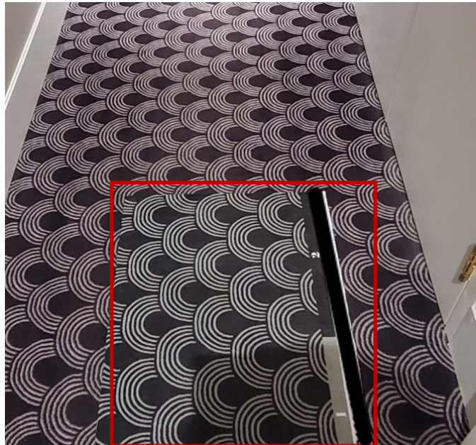
Custom carpet installed in a corridor. The approved strike offs are laying at the foot of the photo in red square. Is this a color match? Is it possible the color was matched under different lighting in manufacturing to installation?
