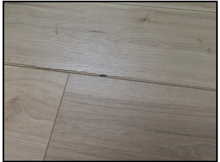
Broken tongue edge of rigid core click/floating flooring due to flexing from traffic
