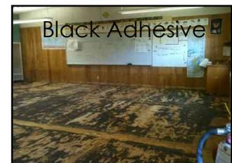
The proper way to remove the adhesive is detailed in the RFCI (Resilient Floor Covering Institute) "Recommended work practices for removal of resilient floor covering."
