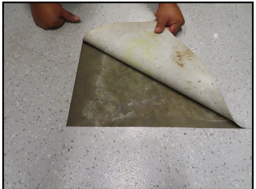
Flooring installation failure over Type 1L concrete
