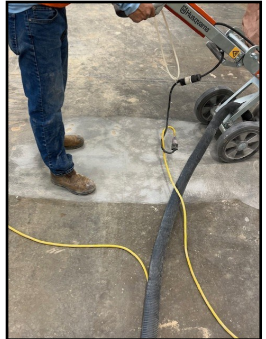
Odd appearance of this Type 1L concrete substrate
